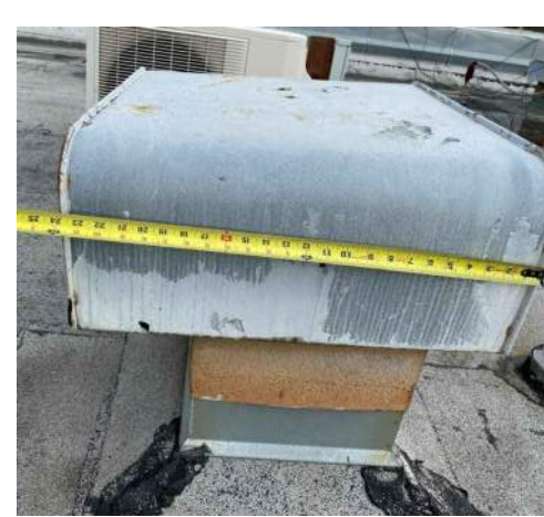
27. Powered Vent Cap Type 1F - Exhaust - Exst
