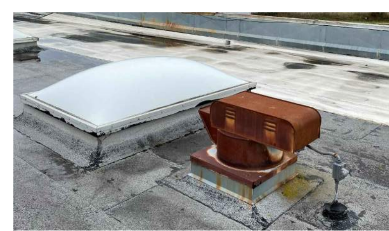
24. Powered Vent Cap Type 1C - Exhaust - Exst
