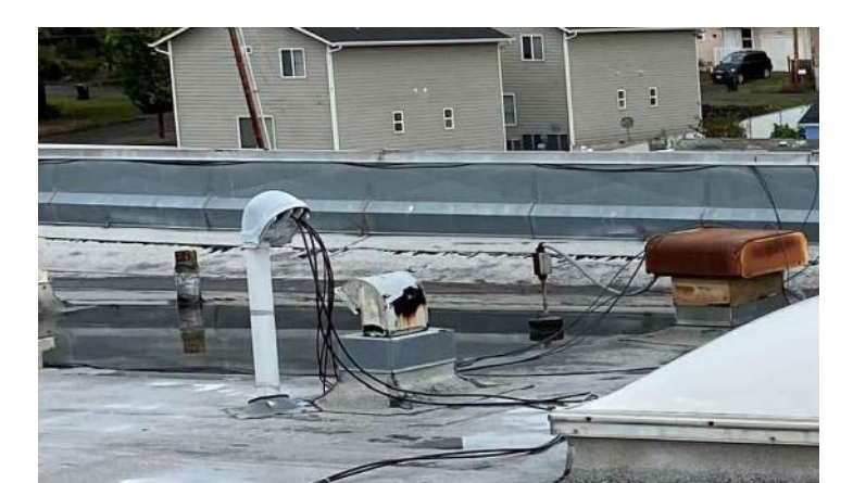
46. Cable Weatherhead
