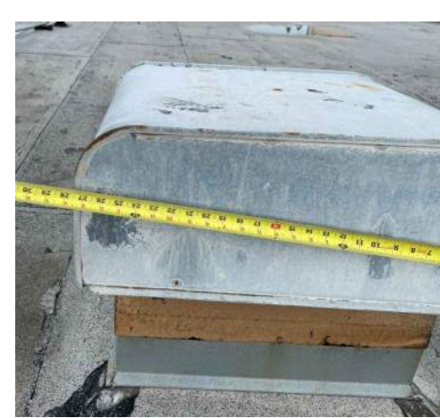
27. Powered Vent Cap Type 1F - Exhaust - Exst
