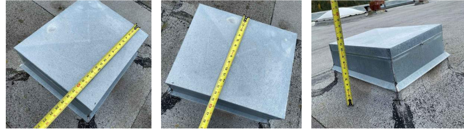
8. Roof Curb Sht Mtl Cap - Exst
