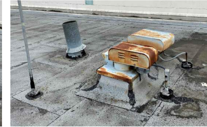
26. Powered Vent Cap Type 1E - Exhaust (Small) - Exst
