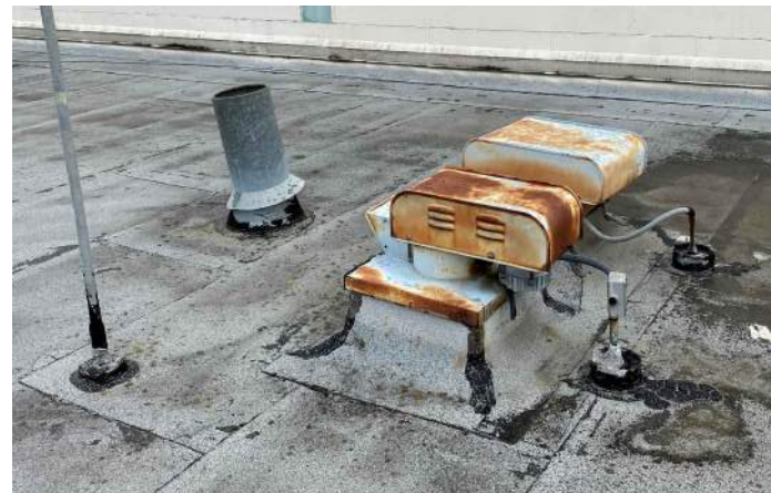
26. Powered Vent Cap Type 1E - Exhaust (Small) - Exst
