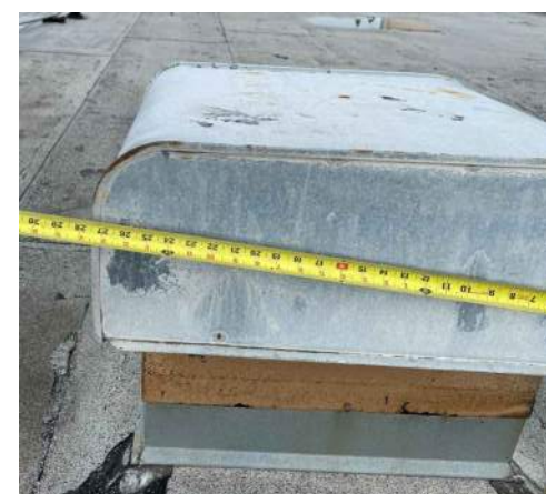
27. Powered Vent Cap Type 1F - Exhaust - Exst
