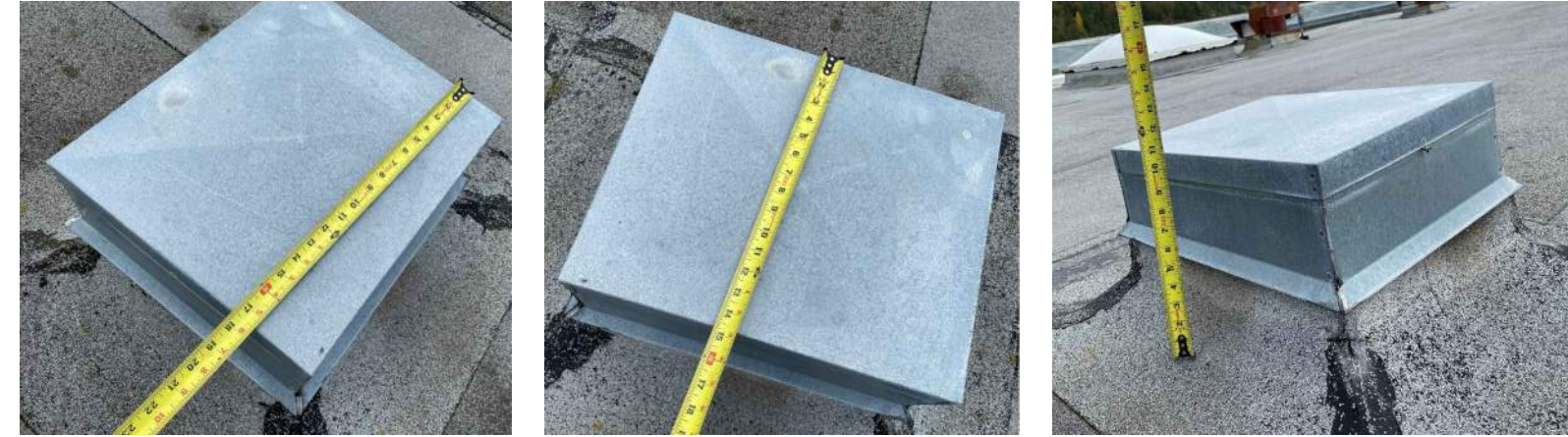
8. Roof Curb Sht Mtl Cap - Exst
