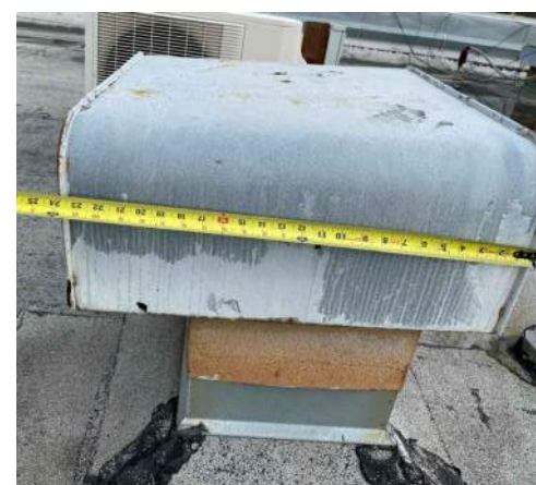
27. Powered Vent Cap Type 1F - Exhaust - Exst
