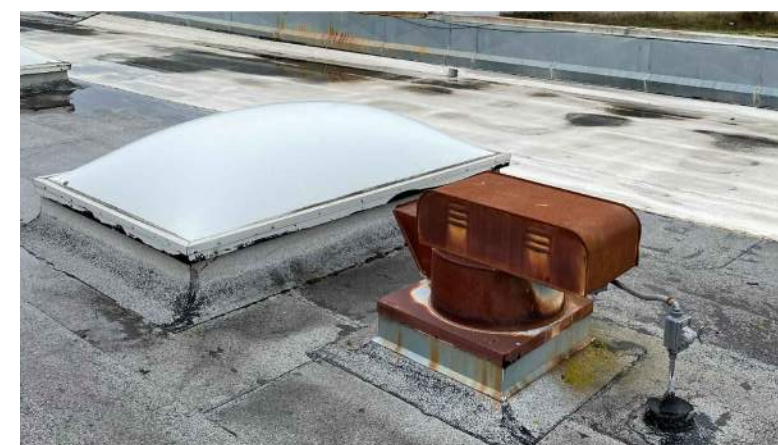
24. Powered Vent Cap Type 1C - Exhaust - Exst
