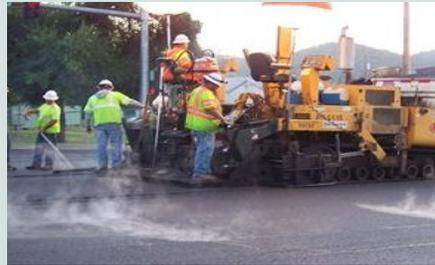
The City is currently out to bid with this year's annual project to maintain the City's street infrastructure. The City is contracting for slurry seals and overlays. A slurry seal is a very thin layer of aggregate with an asphalt emulsifier applied to a paved surface. Slurry seals are used primarily as preventative maintenance to prolong the life of the paved surface. An overlay is the installation of additional asphalt (usually 1 ½ - 2 inches) over the existing asphalt surface.
